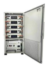
system, high voltage box, power distribution unit, temperature control ...
